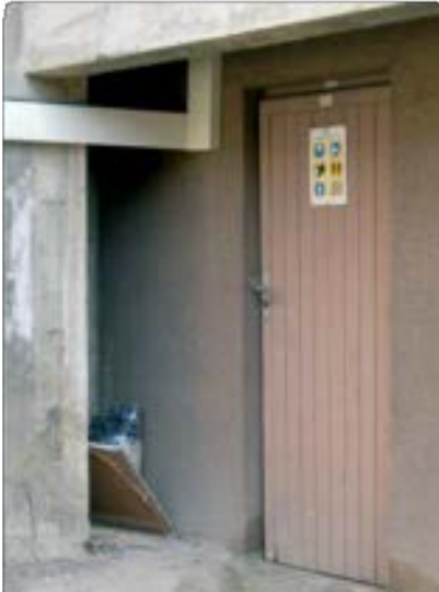
To access the service galleries, the safety instructions must be respected.
