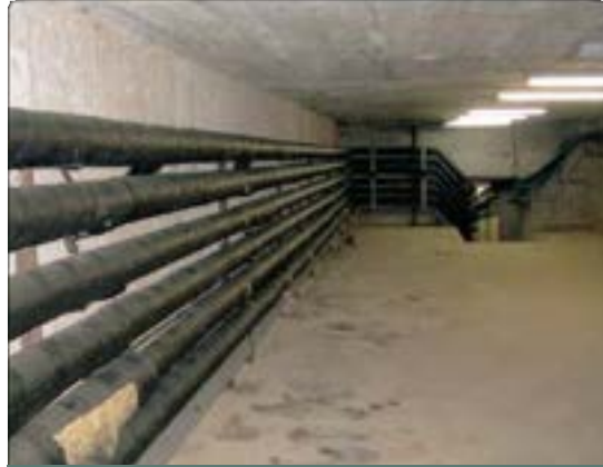
Confined spaces. Galleries.
