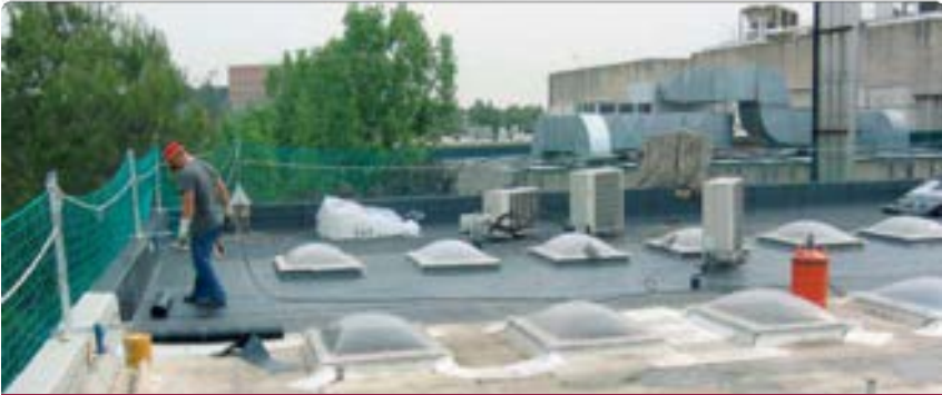
Collective protection takes priority over individual safety when working on roofs.
